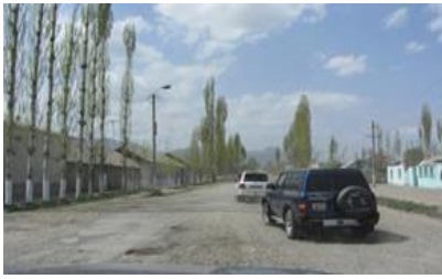
OBI road (Section 28-75)
