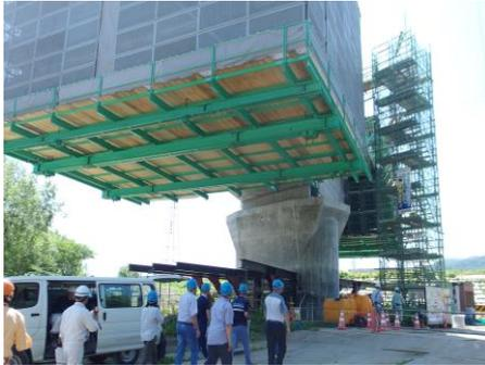
The method of lifting is used in the erection of the overpass near the city of Furano.
